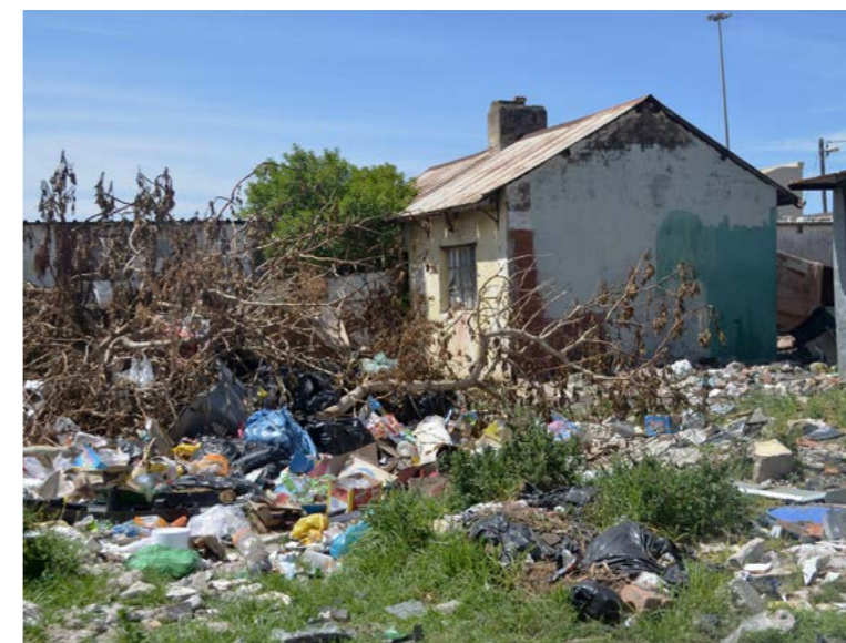
Rubbish piling up in unused corners
