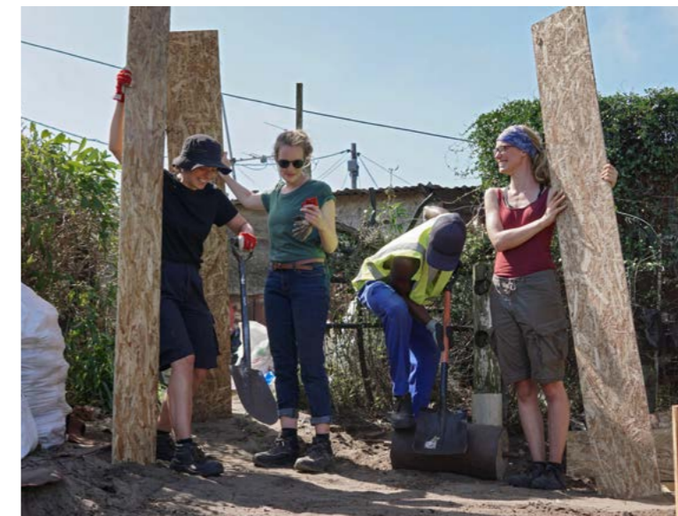
Preparing for the concrete delivery
