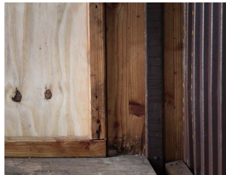
Detail of the interior wall
